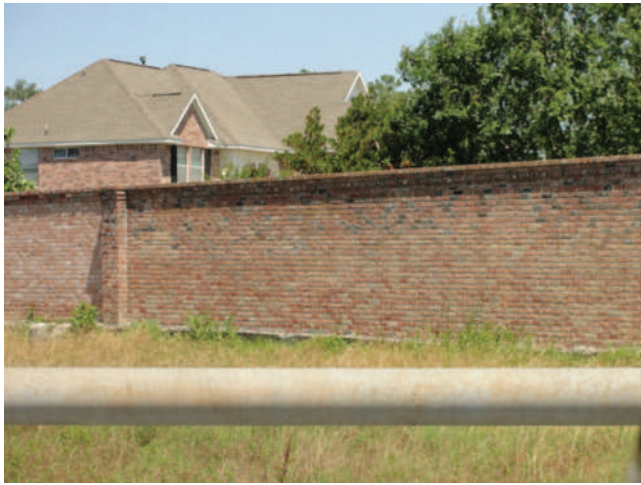
FIGURE C15.6-4 Typical Masonry Ground-Supported Cantilever Wall
