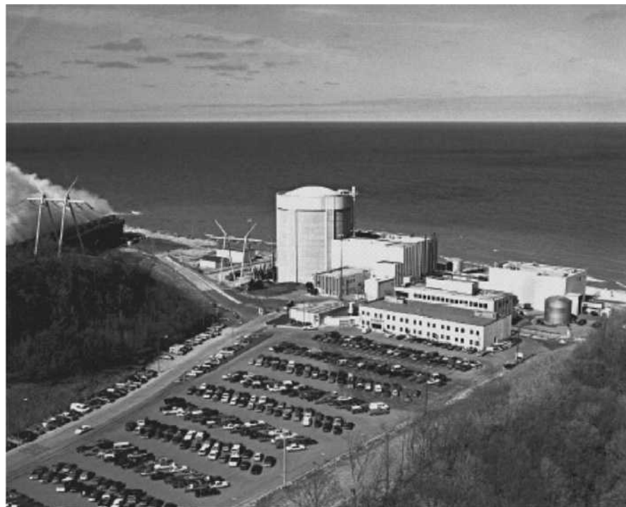
FIGURE C26.7-7 Exposure D: A Building at the Shoreline (Excluding Shorelines in Hurricane-Prone Regions) with wind Flowing over Open Water for a Distance of at Least One Mile. Shorelines in Exposure D Include Inland Waterways, the Great Lakes, and Coastal Areas of California, Oregon, Washington, and Alaska
