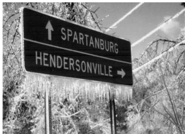
FIGURE C10.2-1 Glaze Ice Accretion Caused by Freezing Rain
