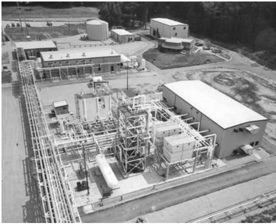
FIGURE C15.1-2 Steel pipe rack
