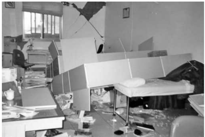
FIGURE C13.1-4 Topped Storage Cabinets
