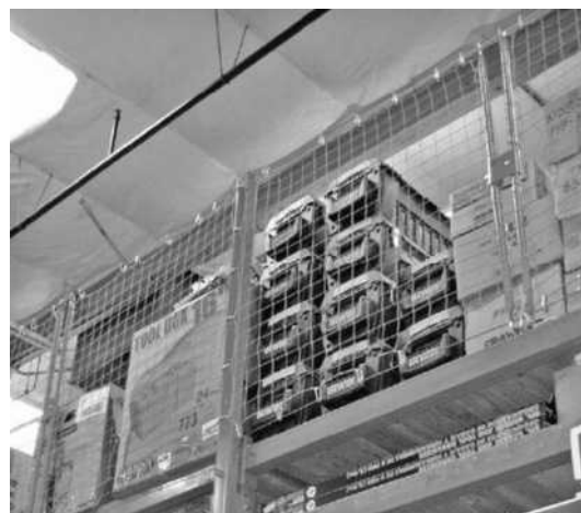
FIGURE C15.5-1 Merchandise restrained by netting
