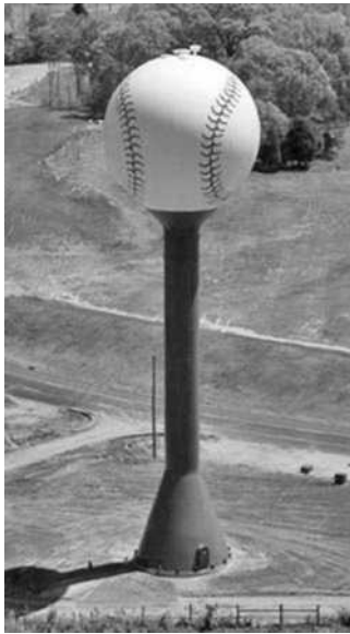
FIGURE C15.7-2 Small-diameter, single-pedestal steel tank
